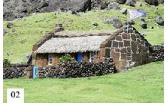
Key: 01 - Old Angelo Saxon house 02 - Old house of the Tristan da Cunha
